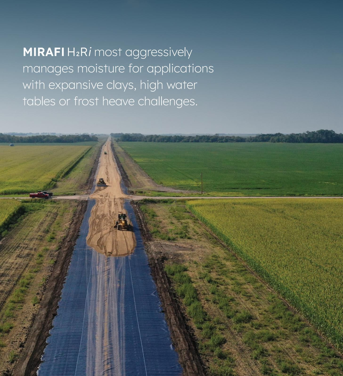
Replacing traditional materials with high-performance woven geotextiles like **MIRAFI H<sub>2</sub>Ri** and **MIRAFI RSi-Series** in unpaved roadways can reduce CO<sub>2</sub> emissions by more than 70%.\*
