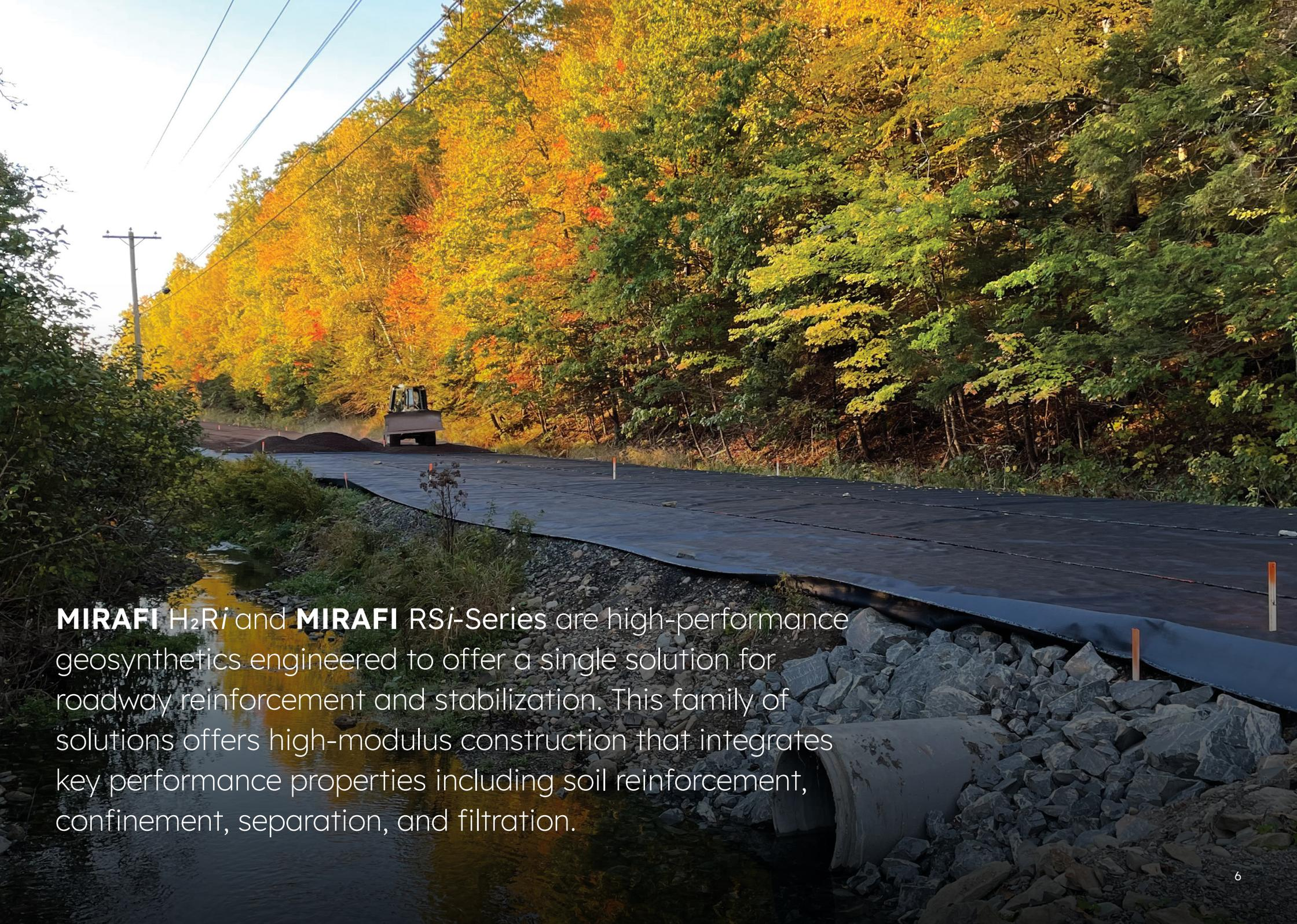
**MIRAFI H<sub>2</sub>Ri** and **MIRAFI RSi-Series** are high-performance geosynthetics engineered to offer a single solution for roadway reinforcement and stabilization. This family of solutions offers high-modulus construction that integrates key performance properties including soil reinforcement, confinement, separation, and filtration.
