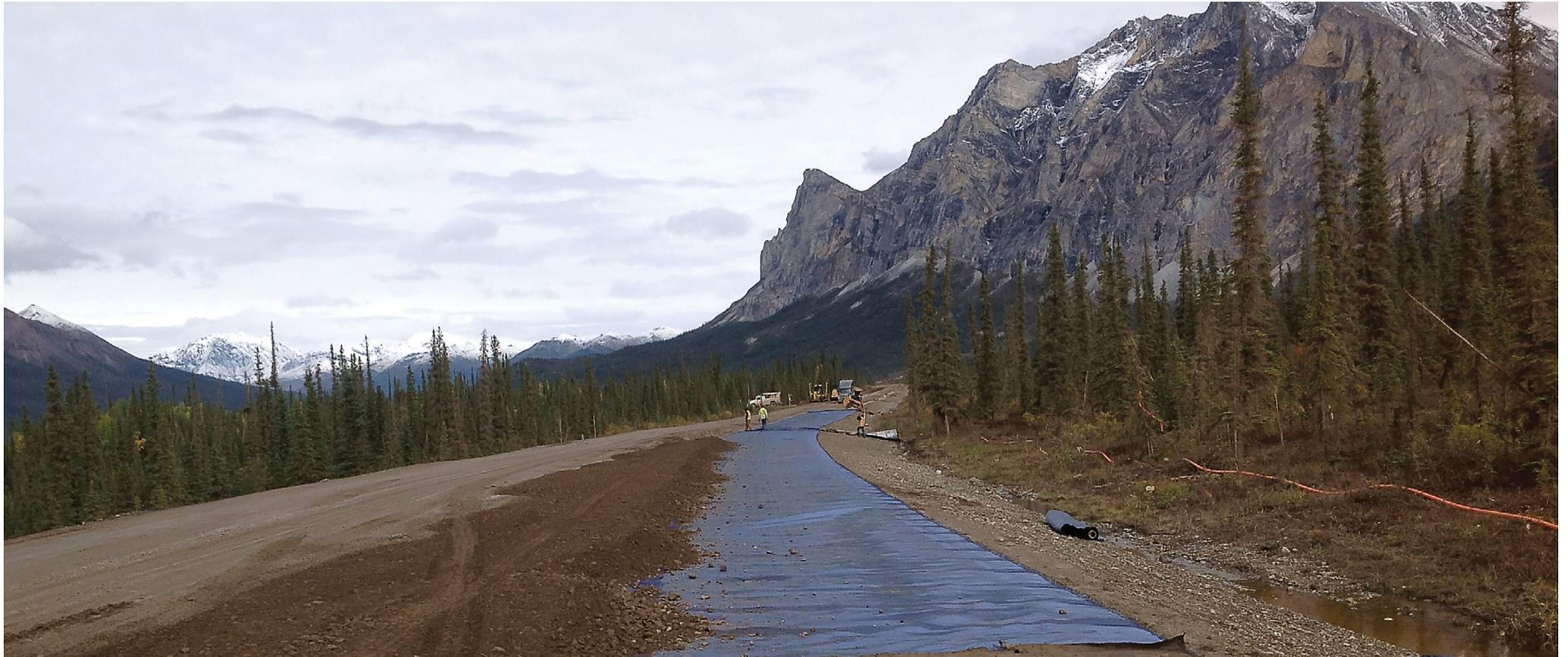
Water is the biggest threat to the performance and durability of roadway infrastructure. To mitigate its damaging effects, Solmax has engineered **MIRAFI**® H<sub>2</sub>Ri and RSi-Series, offering a range of moisture management solutions for base course reinforcement and subgrade stabilization.
