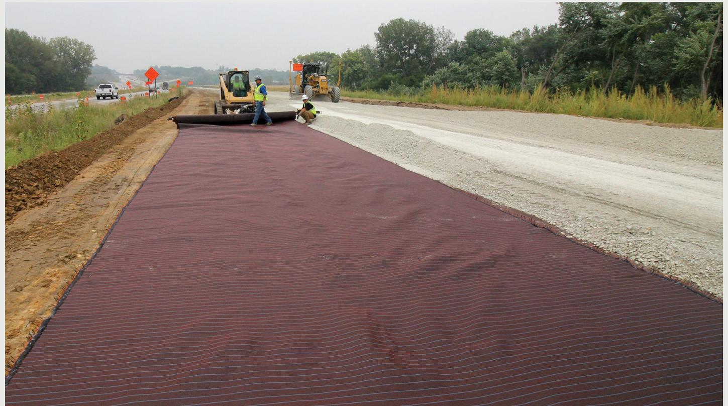
Perched water below roadways will weaken the subgrade leading to damage including potholes and rutting. Using a geosynthetic with moisture management is an effective way to mitigate these issues in both paved and unpaved roadways.
